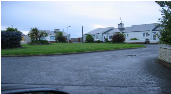
St Mary’s Park Group Housing Scheme, Dunsink Lane, Dublin 10
